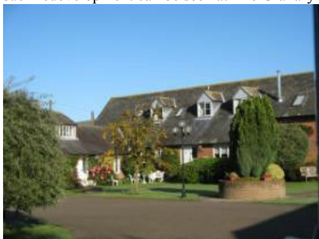
Redundant farm building redeveloped for housing at The Granary
